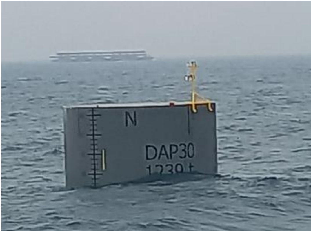
Figure 3: Photograph of installed Monopile showing temporary Aid to Navigation Marking
